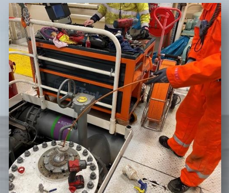
Offshore valve inspection
